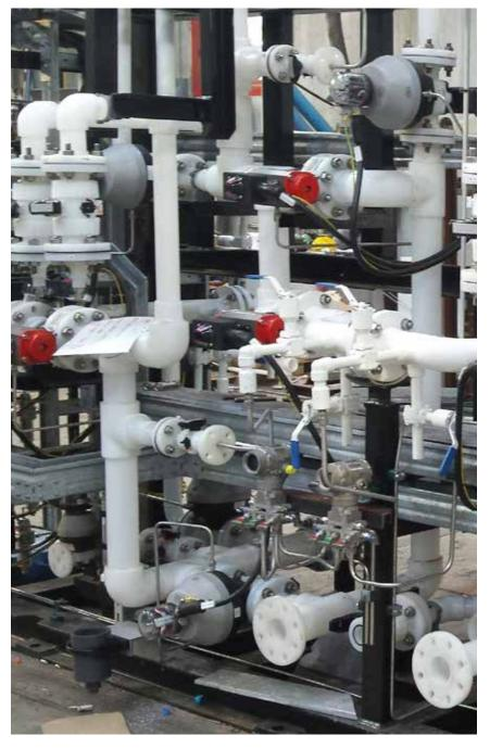
The FIP PVDF system is the best alternative to metal materials due to its high purity and exceptional chemical and mechanical performances over a wide range of temperature.
