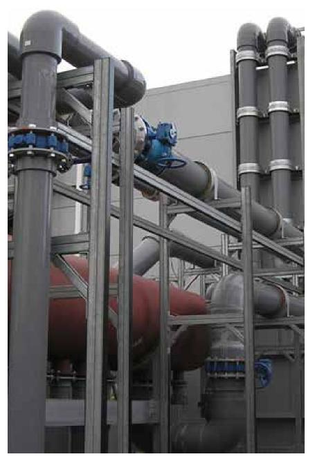
SuperFlo ABS is a high performance chilled and cold water system, solvent a solvent welded, fully matched pipework system incorporating pipe, fittings and valves that is available in both imperial and metric sizes.
