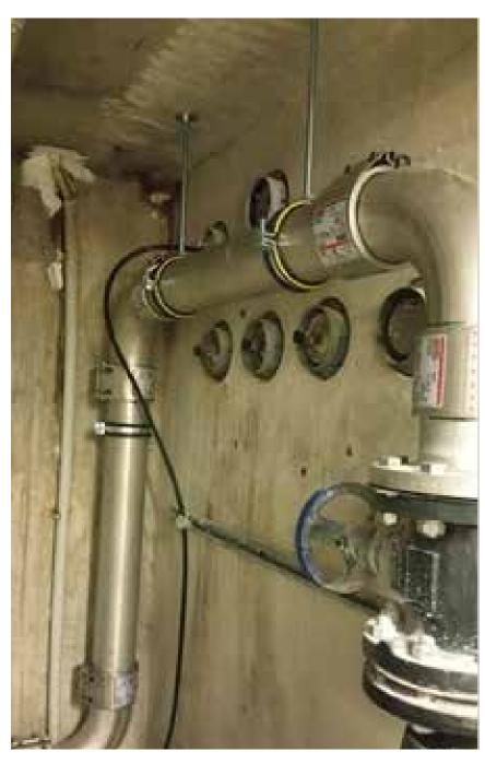
The quick, easy and reliable Straub mechanical joint is an alternative to welding or flange connections.
